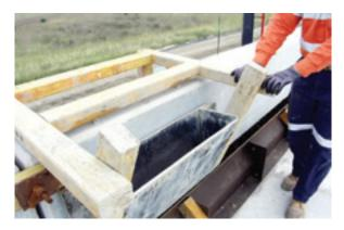
BMD implemented three innovations including a moveable stich pour formwork system to pour concrete parapet stiches
